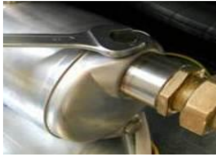
Picture 15 – Pump purging
