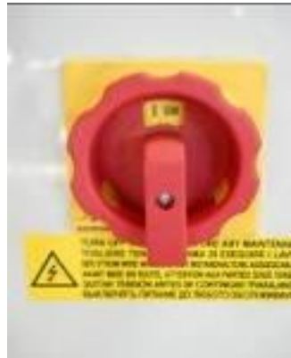
Figura 16 – Interruptor general en ON
