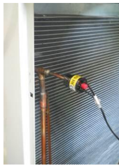
Pressostat haute pression
