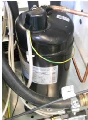
Picture 21 – Compressor placement
