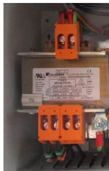
Picture 6 - Unit CE: Factory setting 400/3/50
